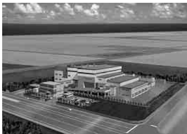
Fig. 1 Mizushima eco-works plant
